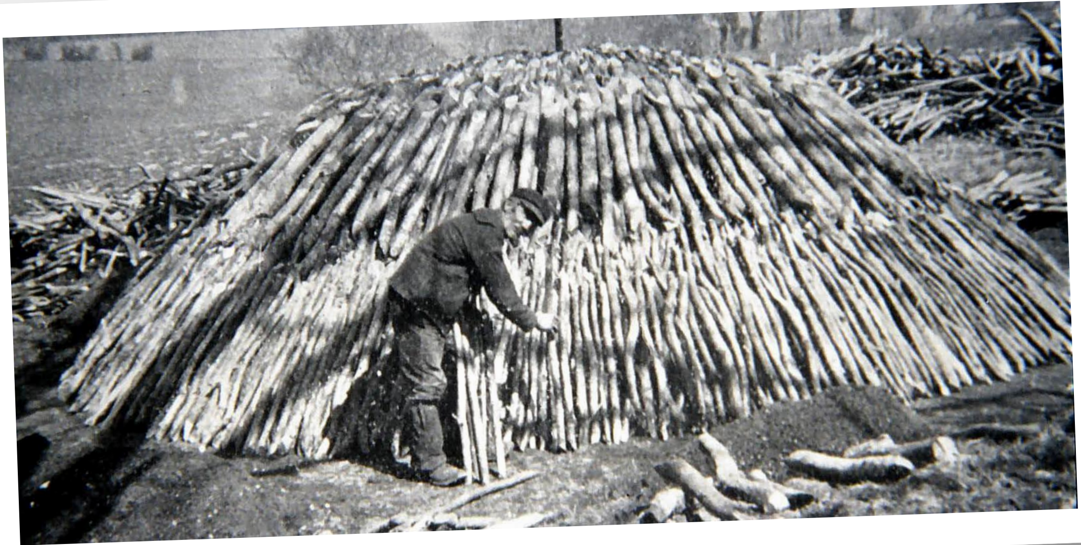
Jim Smith of Manor Cottages, Sedlescombe's Charcoal burner in the start of the 20 th century setting up the stack of wood for slowly charring over several days in Petley Wood
